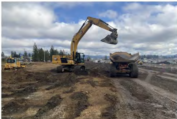
Photos showing relocation of structural fill material from Areas 18/19 to Phase 3
