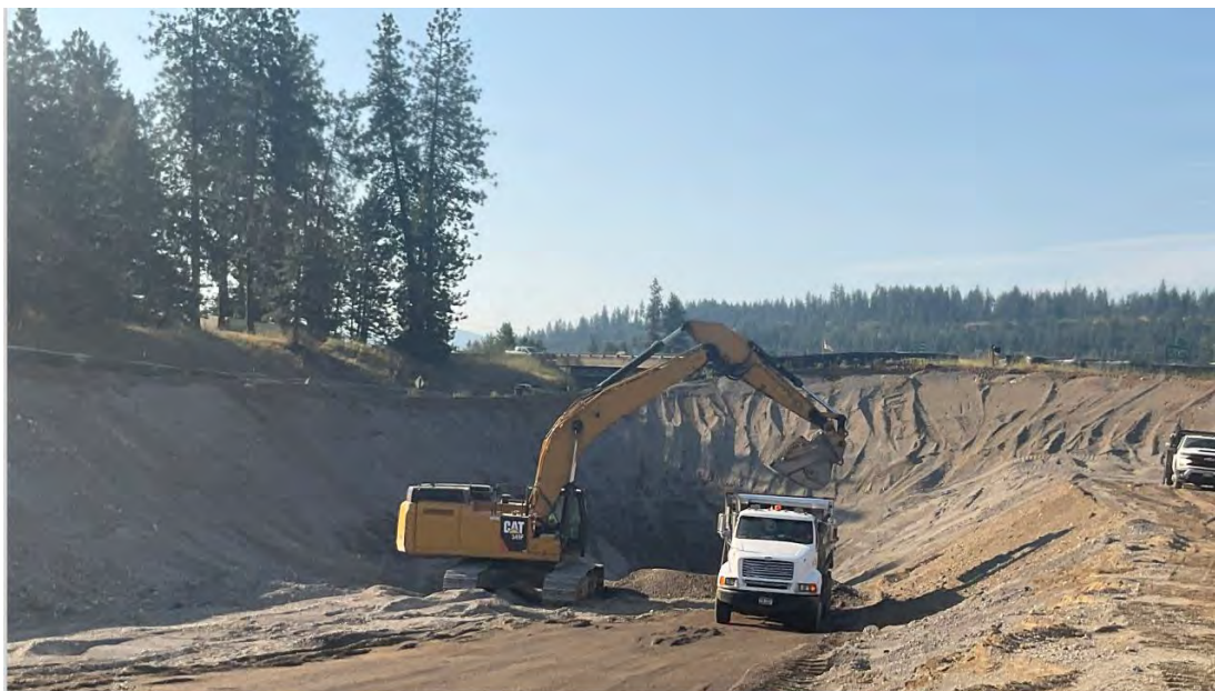
Photo of structural fill material extraction work at Atlas Road borrow site.
