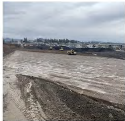
Photos showing relocation of structural fill material from Areas 18/19 to Phase 3
