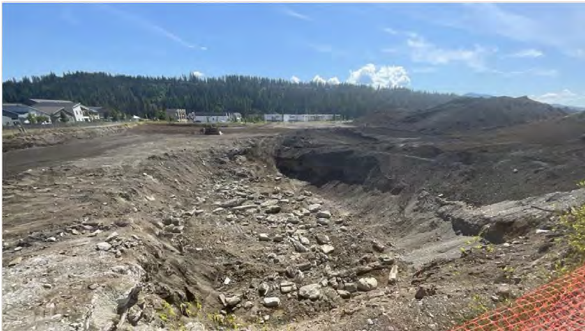
Photo illustrating consolidation of larger scale structural fill material well below final grade on the Phase 3 site.
