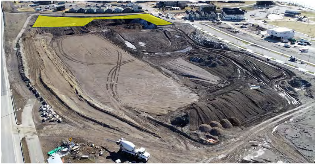
Photo showing the Phase 3 site highlighting in yellow the location of the remaining non-structural fill material.
